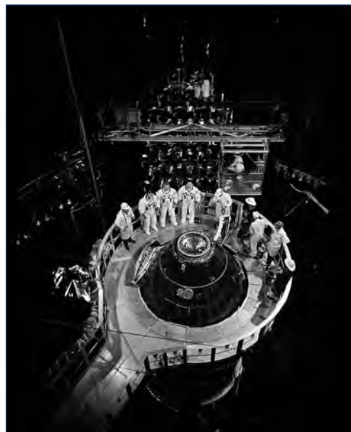
High-angle interior view of Chamber A showing three astronauts preparing to enter the Block II Thermal Vacuum Test Article in 1969. (Image Number S68-37430)
